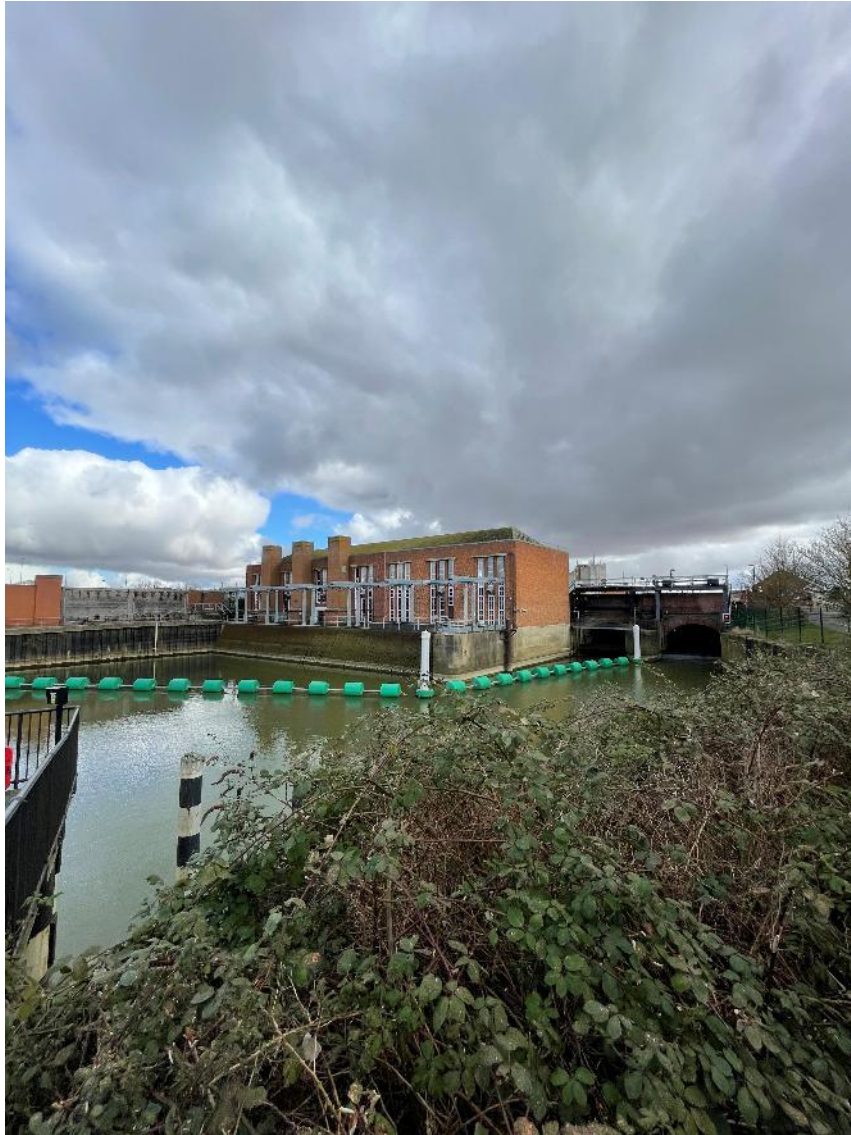
(Photograph 12 – Black Sluice Pumping Station, with sluice gates to the right; facing north-east)
